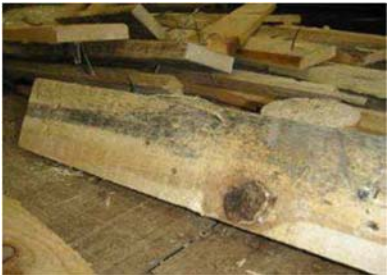
Mold: Not OK
