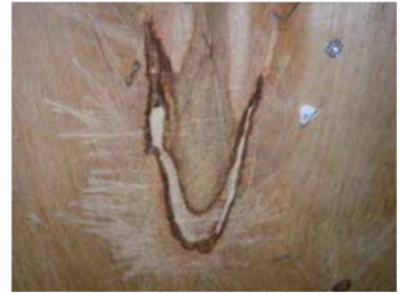
Knot Hole in Plywood: OK
