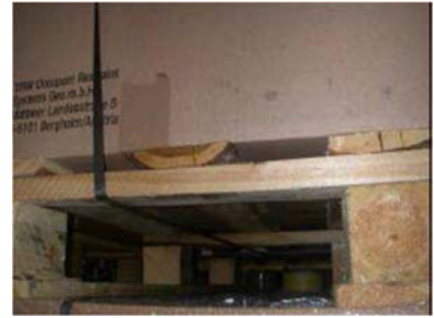
Warped Runners: Not OK
