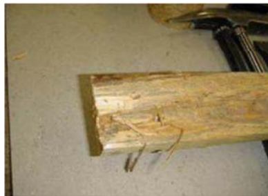
Rotten Wood: Not OK
