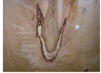
Knot Hole in Plywood: OK
