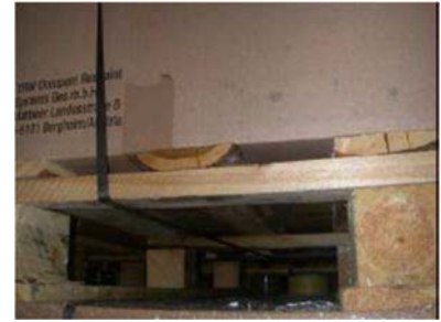
Warped Runners: Not OK
