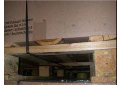
Warped Runners: Not OK
