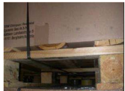
Warped Runners: Not OK
