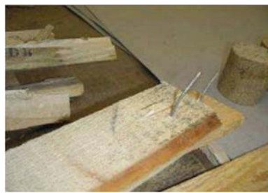
Mold: Not OK
