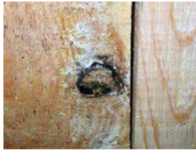
Knot and Mold: Not OK
