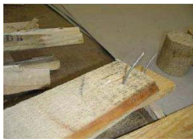
Mold: Not OK
