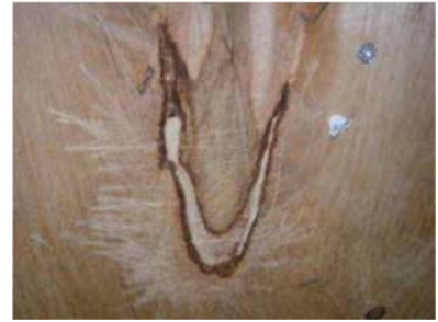
Knot Hole in Plywood: OK
