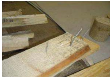
Mold: Not OK
