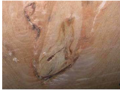
Knot Hole in Plywood: OK
