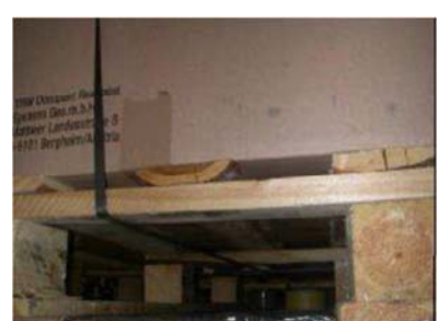
Warped Runners: Not OK
