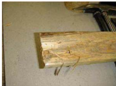
Rotten Wood: Not OK
