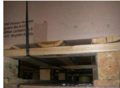
Warped Runners: Not OK
